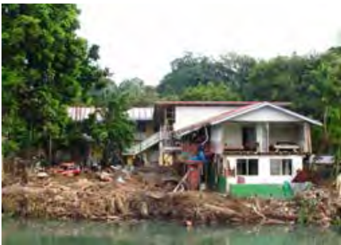
Destruction alongside the Mataniko riverbank in Honiara after flash floods. Photo: Janna Hamilton / New Zealand Red Cross
